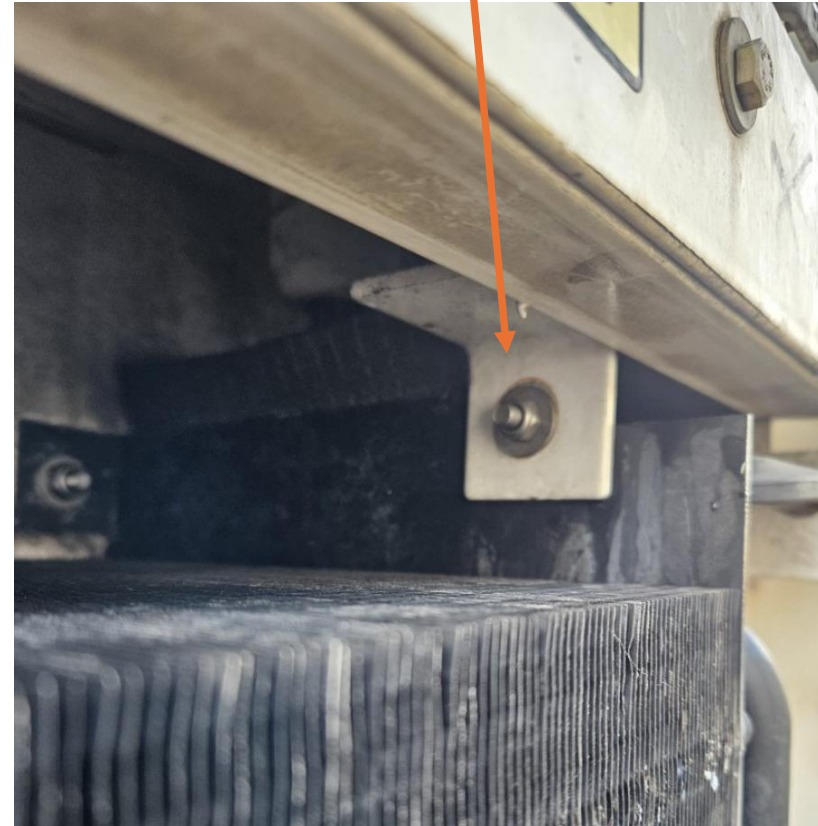
CCB Condenser coil mounting bracket
