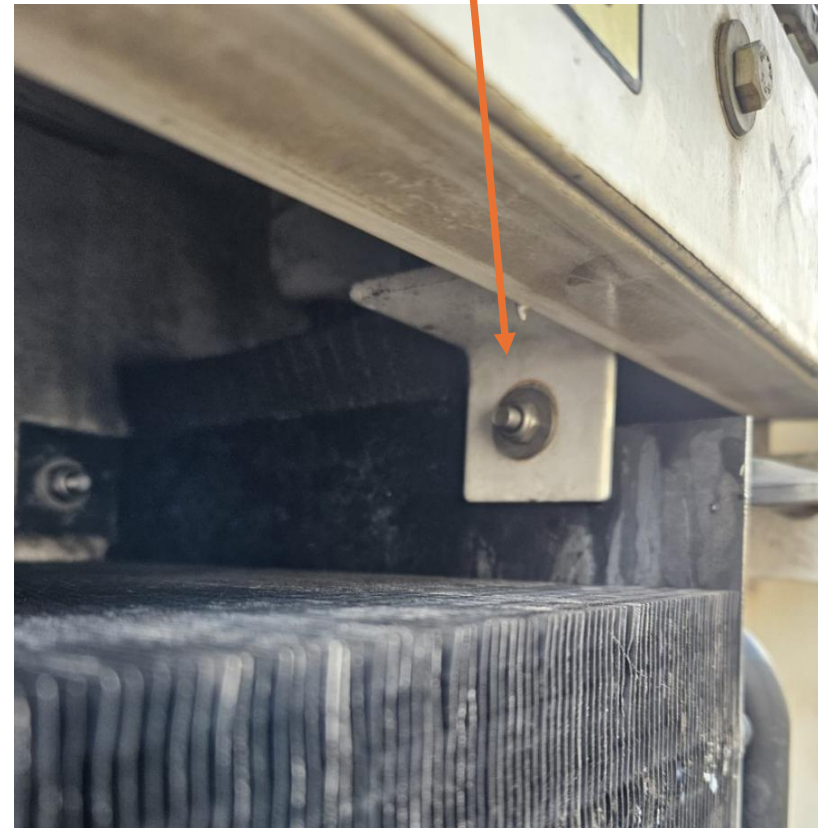
CCB Condenser coil mounting bracket
