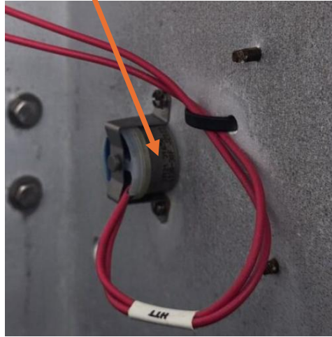
SDT Defrost Termination Switch
